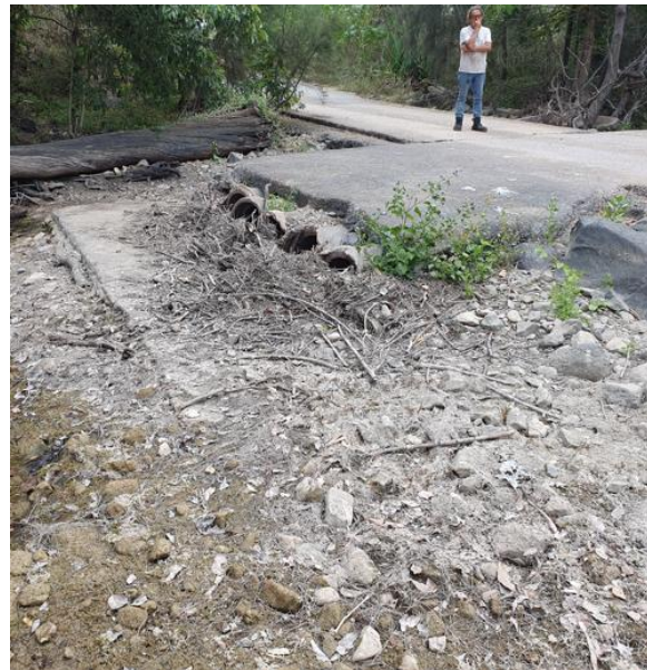
Figure 2 – Culvert causeway
