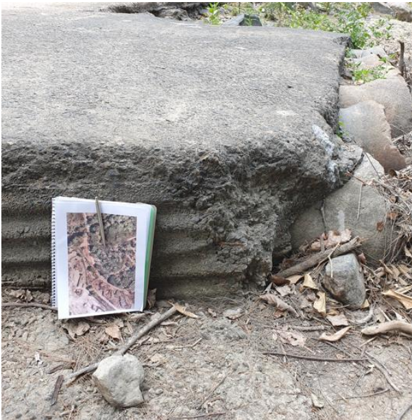
Figure 1 – Depth of concrete over culvert
