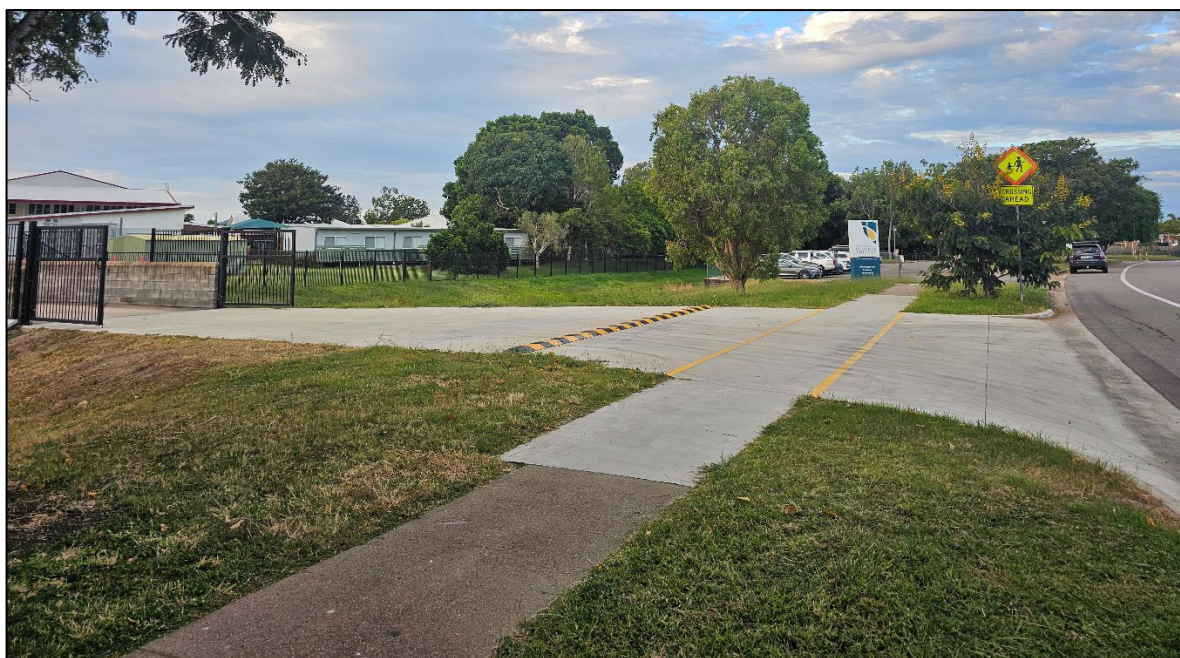
Figure 99. Reconstructed Site access 1 (Looking from the west)
