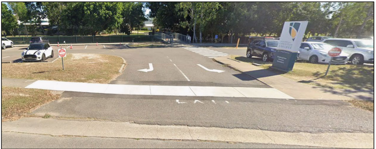
Figure 121. Existing Site access 2 arrangement (Source: Google Street view August 2022)
