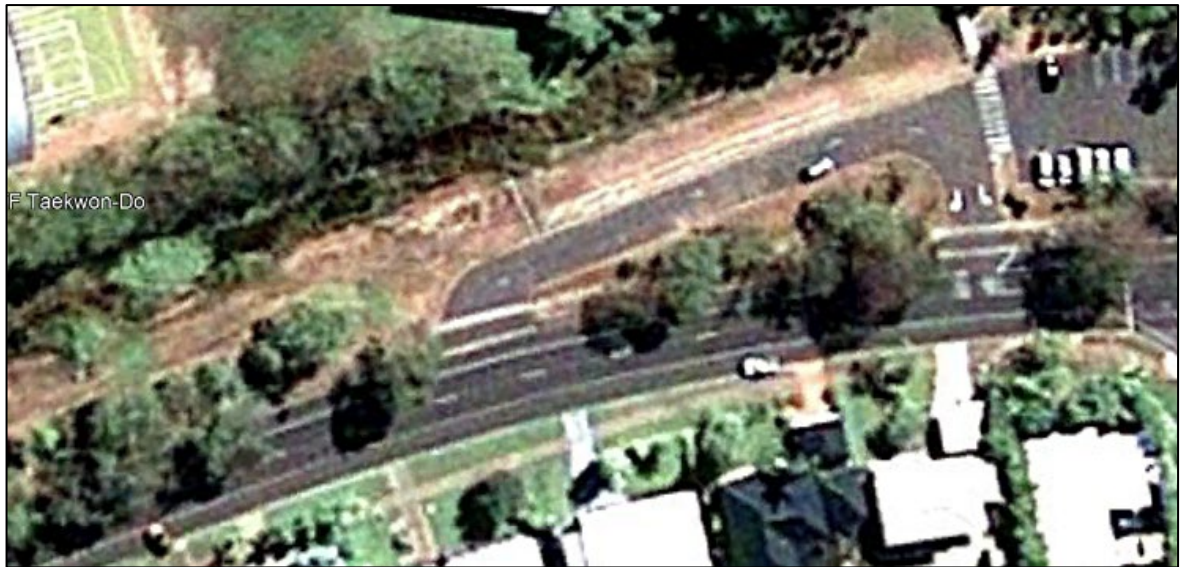
Figure 102. Aerial view of Site access 2 7 October 2007 (Source: Google Earth)
