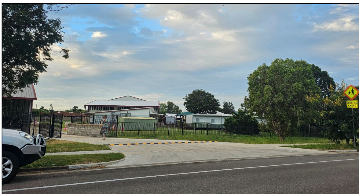
Figure 100. Reconstructed Site Access 1 (looking from across the access)
