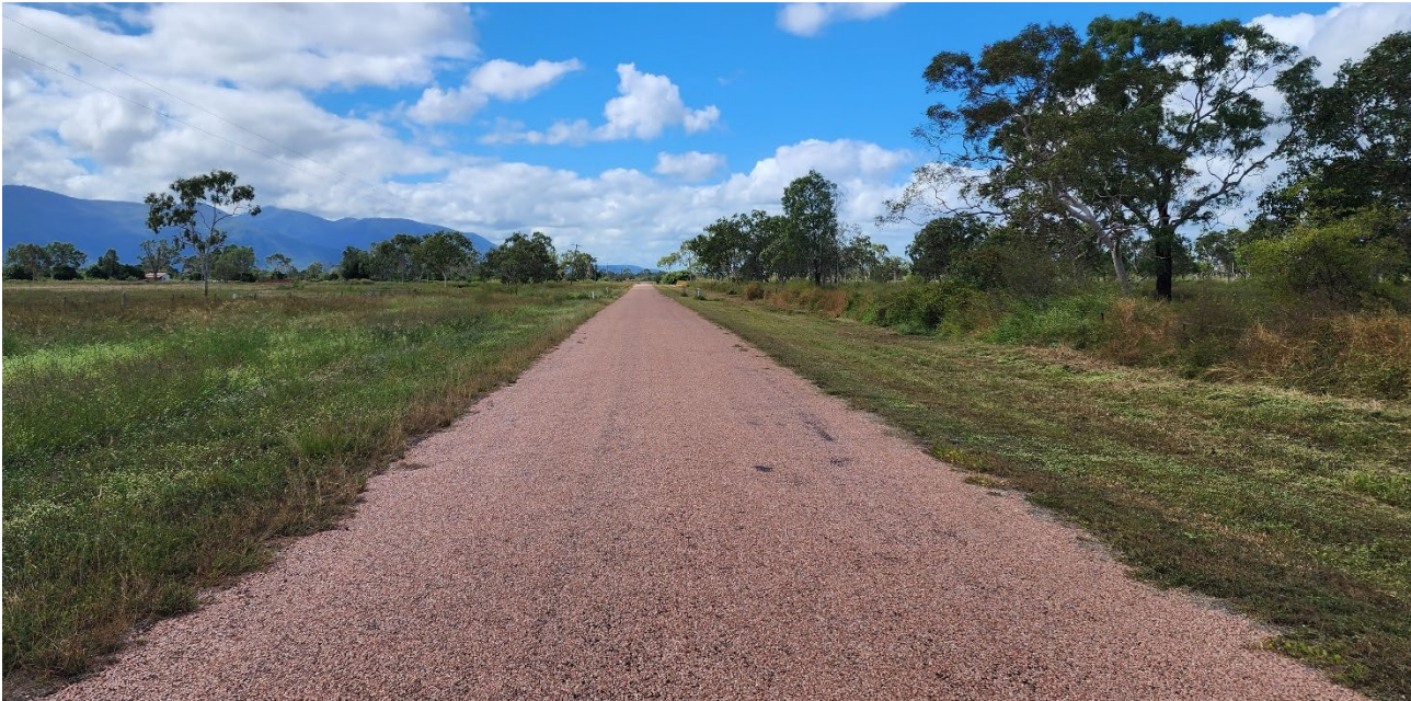
Photograph 4.3 Jones Road facing west near Woodstock Avenue (taken on 14 May 2025)
