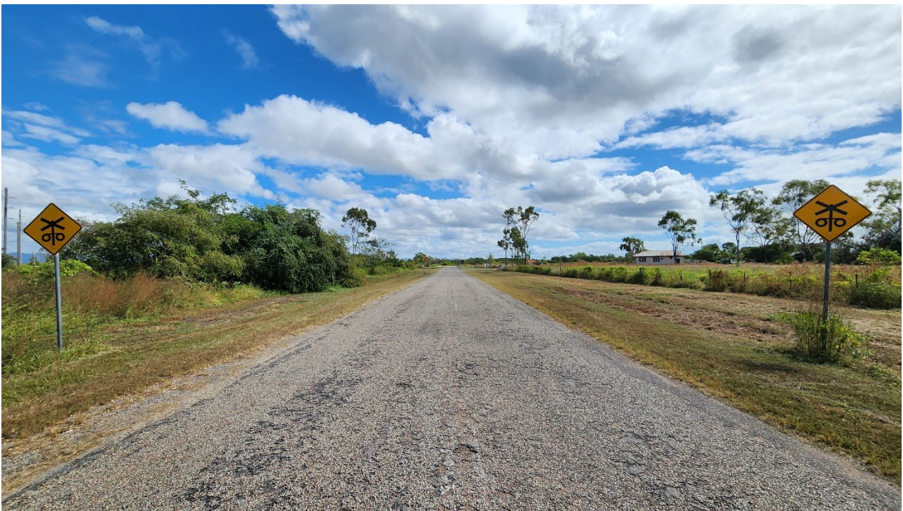
Photograph 4.2 Glenn Road facing west near railway level crossing (taken on 14 May 2025)
