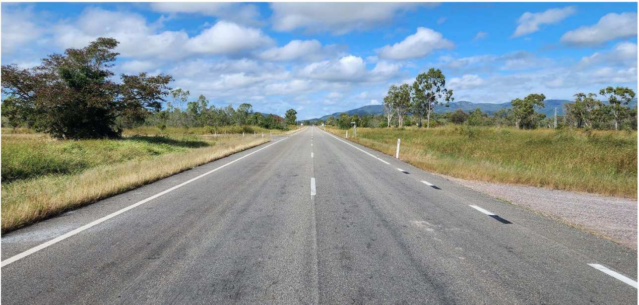
Photograph 4.1 Flinders Highway facing south nearby Bidwilli Road (taken on 14 May 2025)
