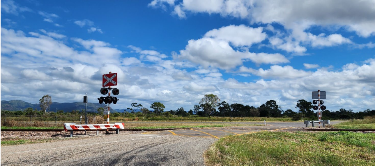
Photograph 4.4 Glenn Road level crossing (taken on 14 May 2025)
