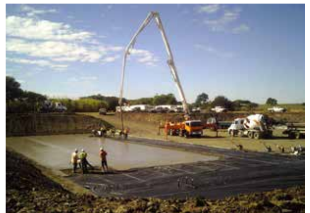
Construction underway: installation of the digester blinder slab at the Rubyanna Wastewater Plant
