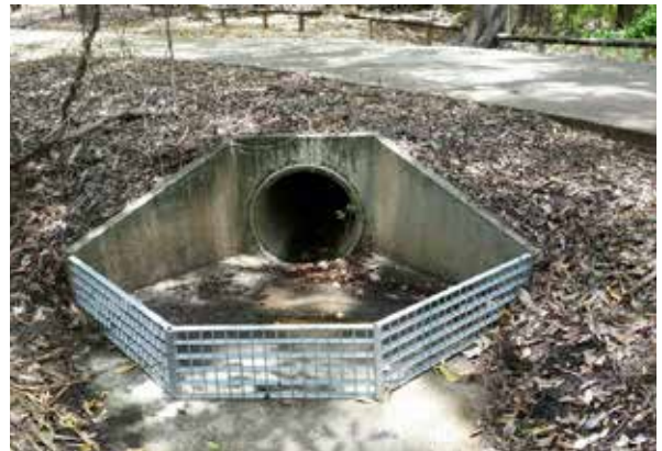
Trapping trash: a pollutant trap installed at Baldwin Swamp Environmental Park
