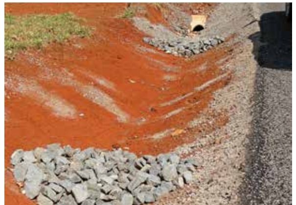
Combatting sediment runoff: sediment control devices installed in a steep roadside drain by council staff
