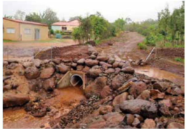
Stormwater slowdown: drain constructed at Hutton Drive, Rangeview, using watershed restoration techniques
