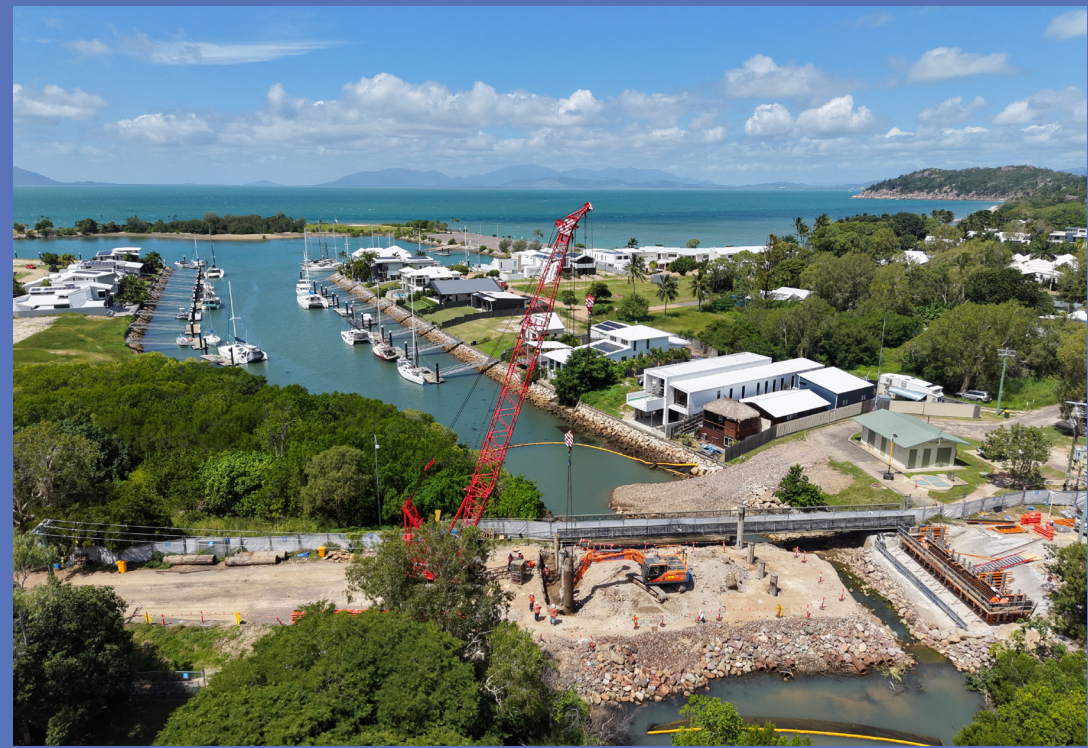
Sooning Street bridge construction
