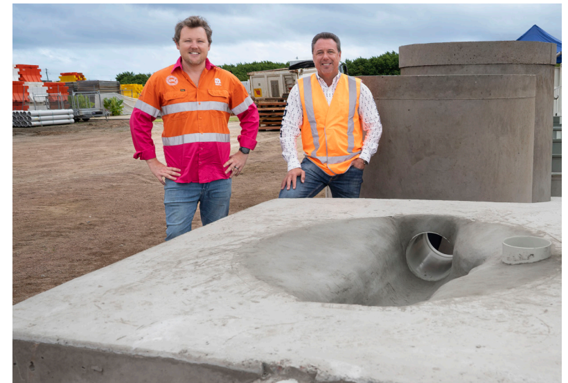
Division 10 Councillor Brady Ellis and Mayor Nick Dametto inspecting a maintenance hole base that will be installed during Stage One
