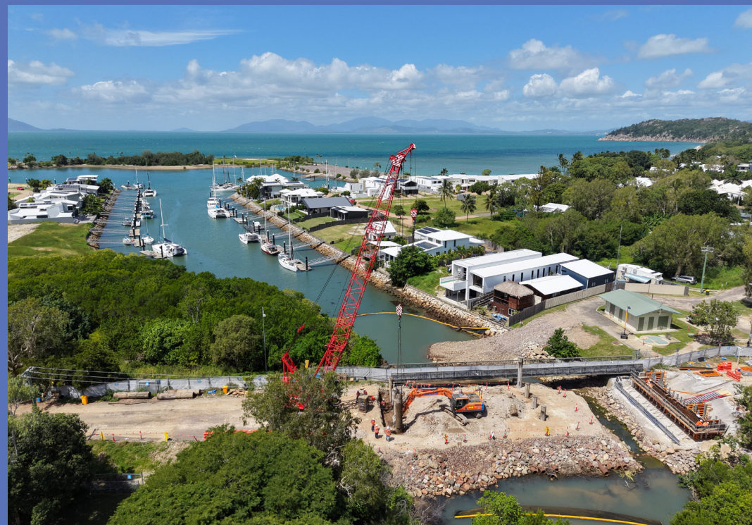
Sooning Street bridge construction
