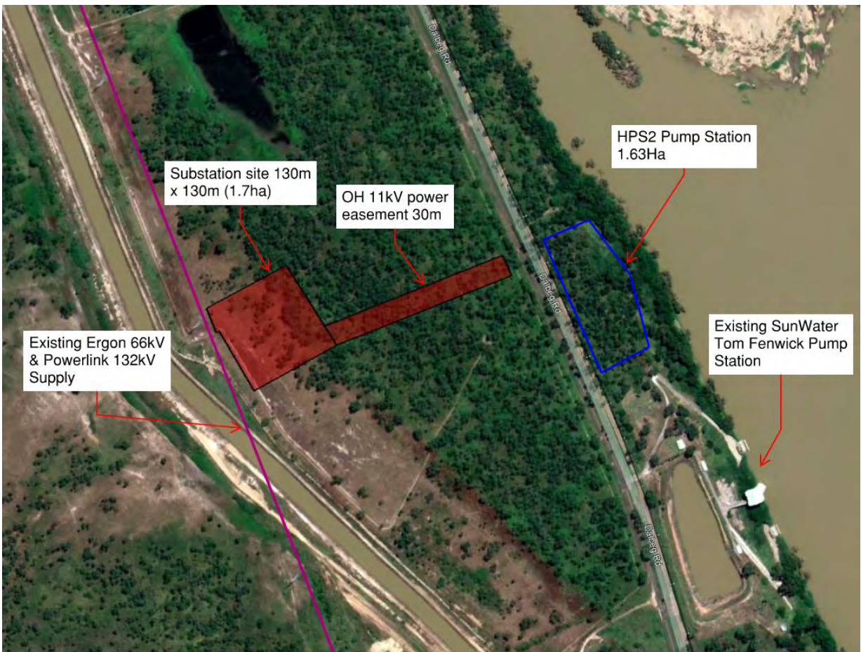
Figure 8 Substation and high voltage power supply
