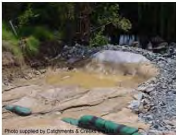
Rock filter dam - geotextile filter
