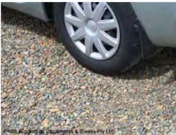
Gravel-stabilised car park
