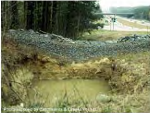
Excavated sediment trap
