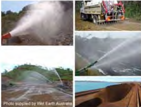
Application of soil binders
