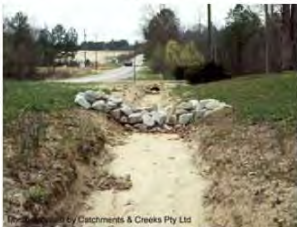
Rock check dam
