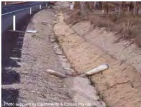
Check dam sediment trap
