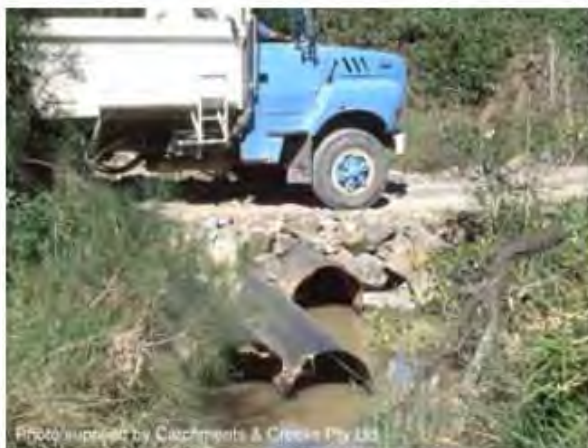
Temporary pipe culvert
