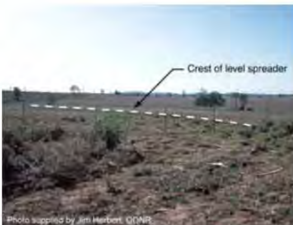
Level spreader used to release road runoff into the adjacent farmland
