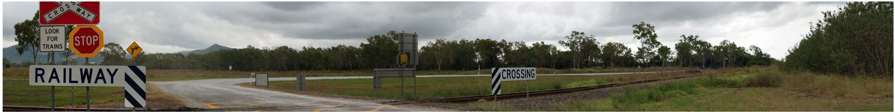
Panoramic view of existing site
