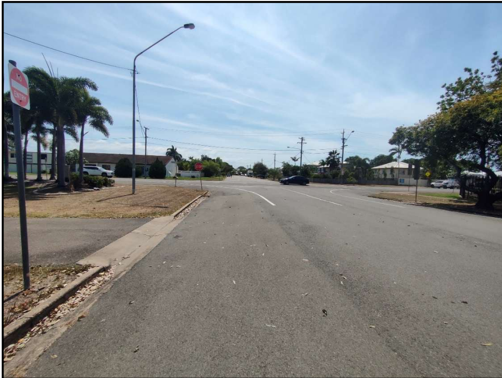
Photograph 1 – Lonerganne Street looking west towards Meenan Street intersection
