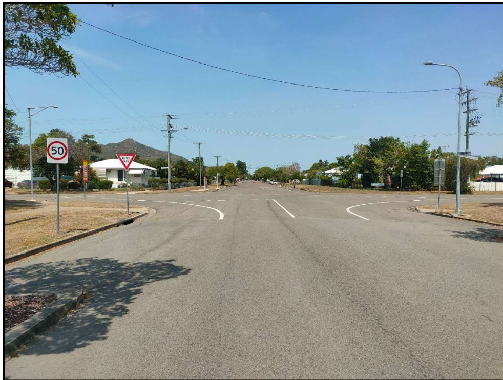
Photograph 5 – Lonerganne Street looking east towards Peel Street intersection
